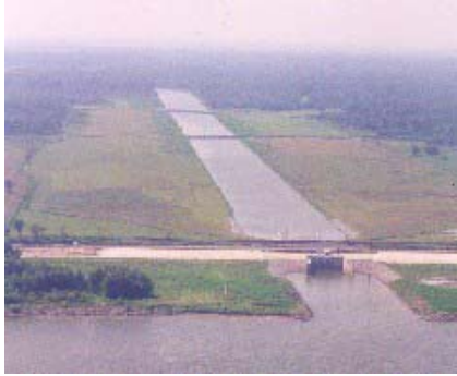
Freshwater diversion canal at Davis Pond.
